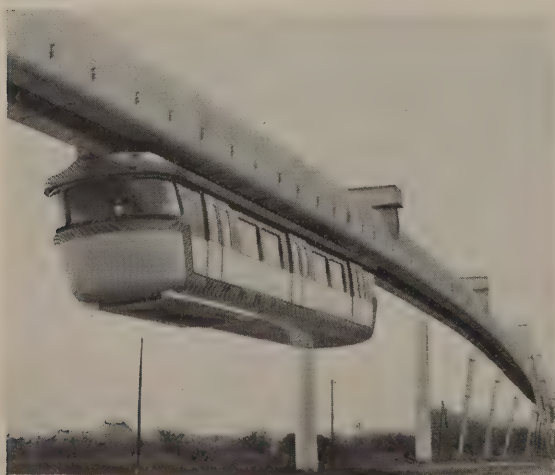
34 The experimental monorail track of S.A.F.E.G.E. TRANSPORT near Paris. The car is suspended from rubber tyred bogies running inside the duct, and operation is thus silent and impervious to weather.
